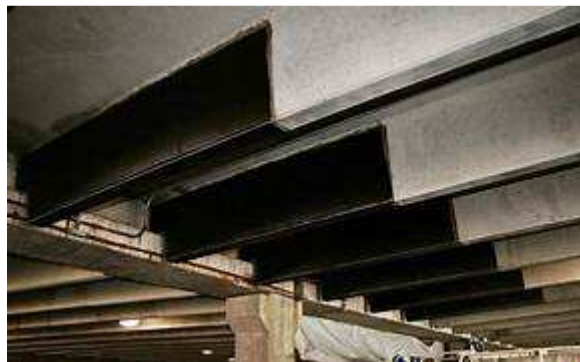
Figure 5: Concrete Beams wrapped with CFRP
