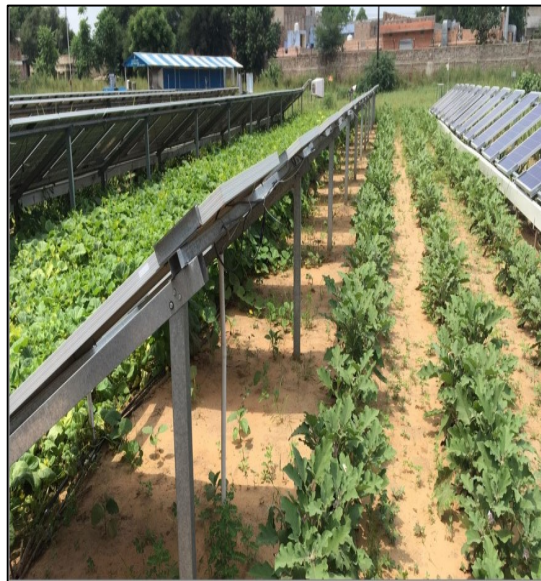
Figure 6 : AV system of 105 kW capacity located at CAZARI (Source: Santra et al. , 2018 [16])
