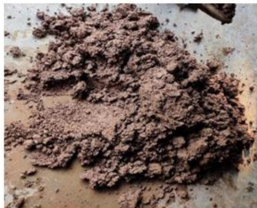
Figure 10: Wet mixing of materials
