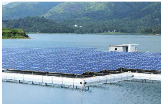
Figure 3: Floating PV System Source: Google Images
