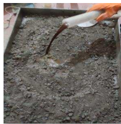
Figure 7 : Super Plasticizers Mixing in Dry State of Concrete
