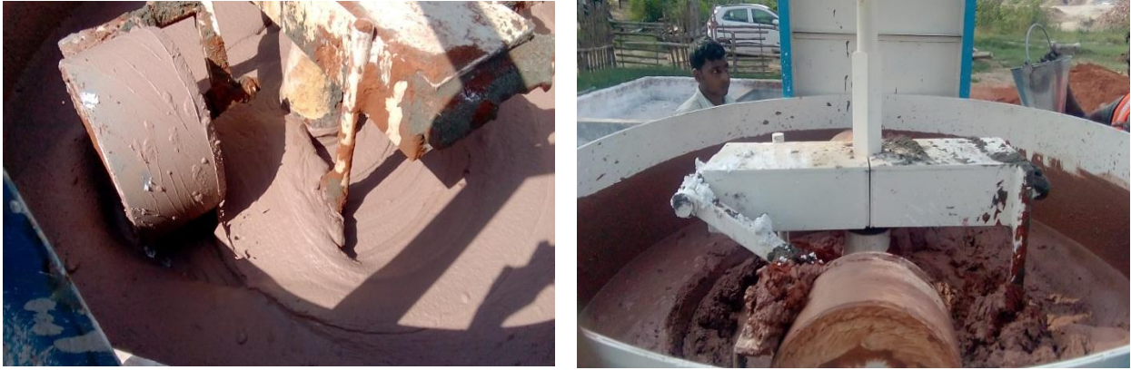
Figure 8: Showing the Preparation of lime mortar- Ratio (1:1:1) -1 Lime: 1 Surkhi: 1 San
