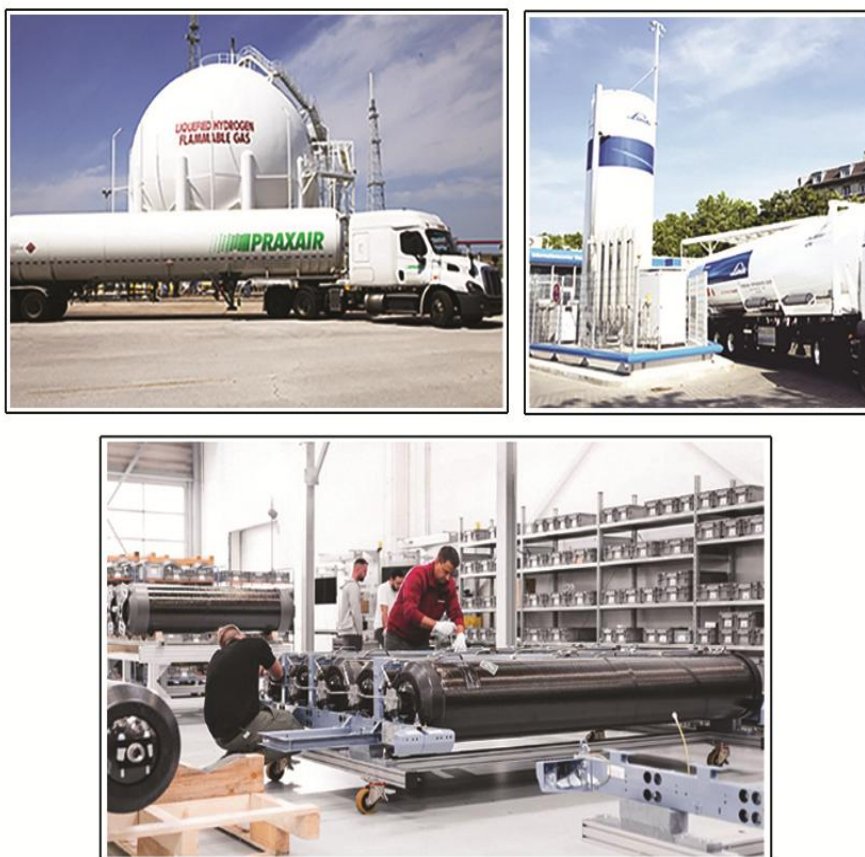
Figure 4: Three Different Liquefied Hydrogen Storage Tanks
