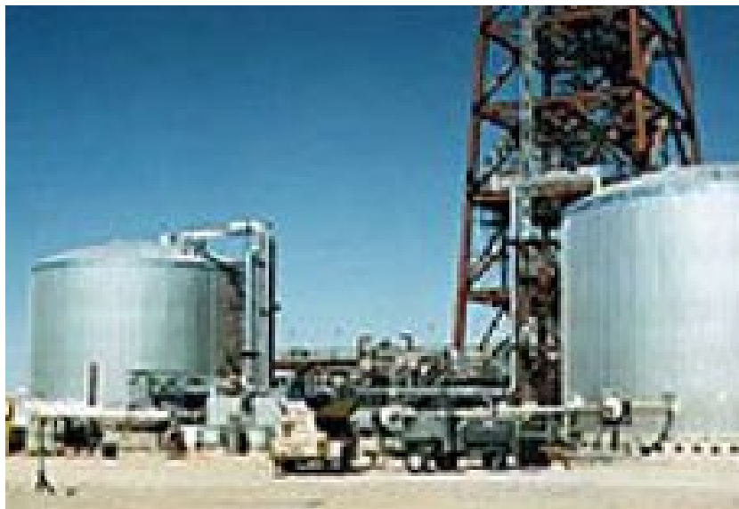
Figure 8: Direct Two-Tank System
