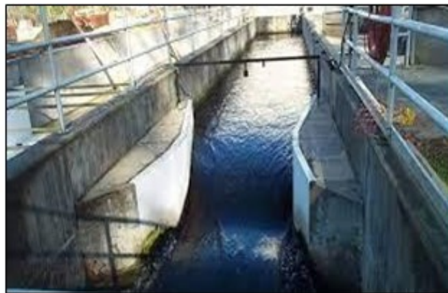
Figure 4: Parshall Flume in Water Drainage Work (Source: https://tracomfrp.com/parshall-flumes-work )
