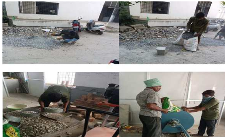
Figure 3: Crushing of Recycled Aggregate
