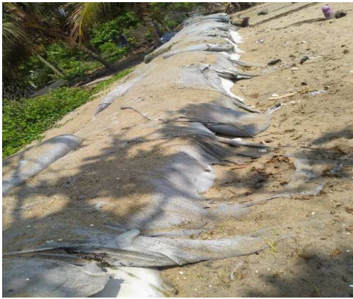
Figure 9: Damaged geobags
