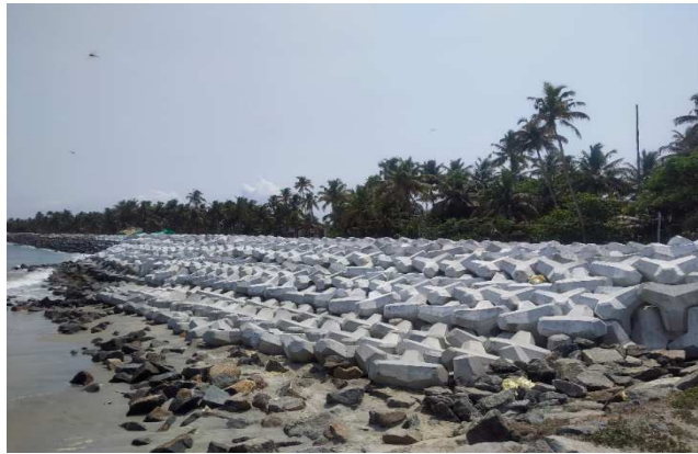
Figure 13: Tetrapod seawall at Chellanam
