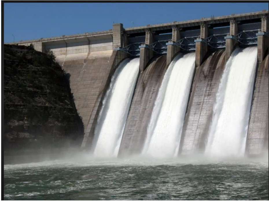
Figure 1: Dam of Hydro Electric Power Plant
