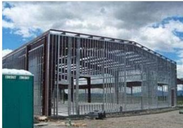
Figure 2: Example of structural design for LGSF Construction
