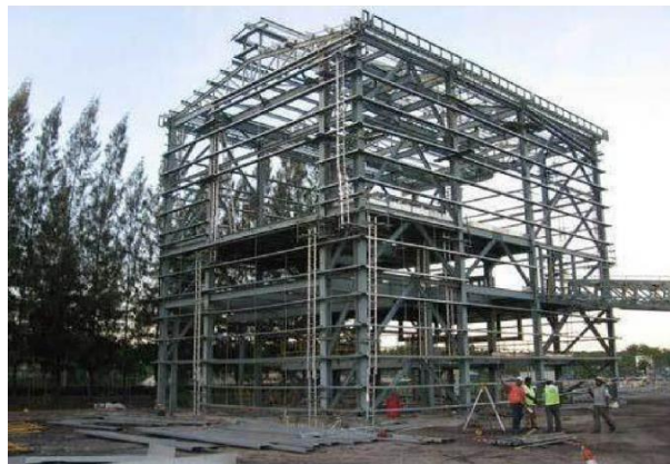
Figure 1: Steel Structure Installation
