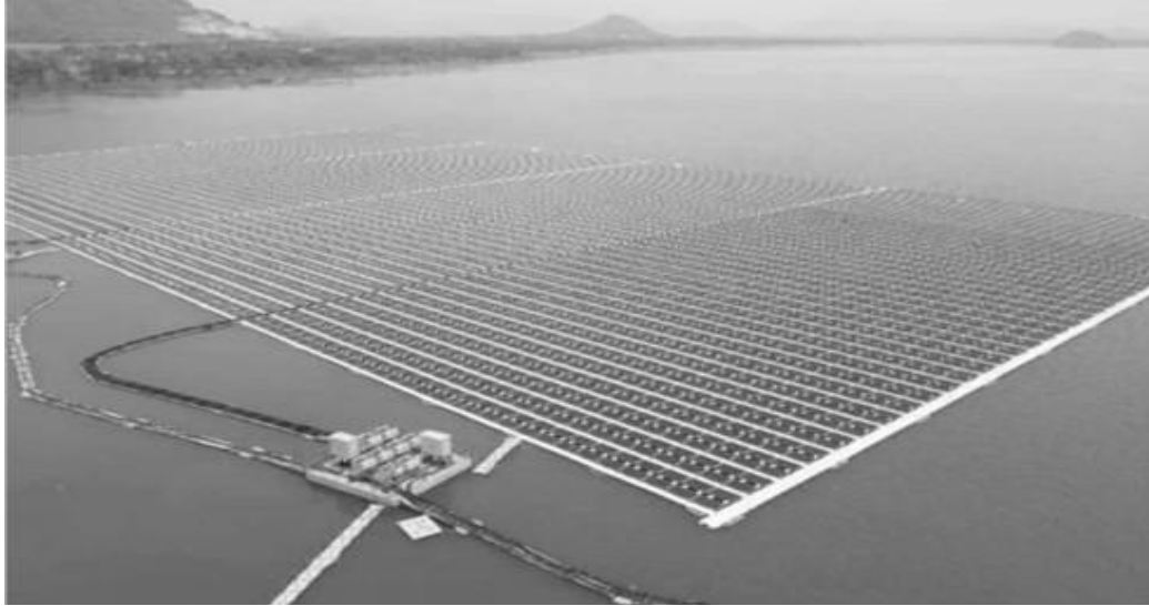
Figure 13: Utility scale FSPV at Ramagundam, India
