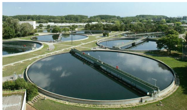
Figure 6: Sewage treatment Plant (STP) at OKHLA (New Delhi- India)
