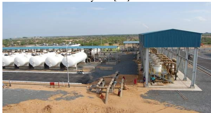
Figure 4: The Minjur Desalination Plant (Tamil Nadu- Chennai, India)
