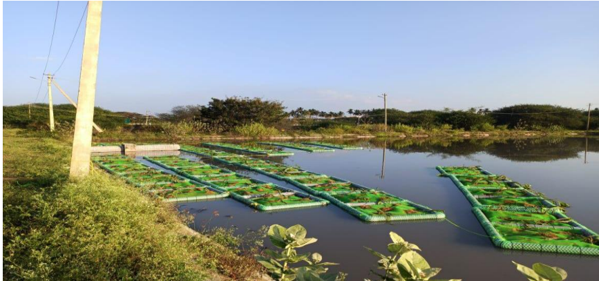
Figure 6: Installed floating wetland in pond (source: Maturation Pond, STP Chikkaballapur, karnataka )
