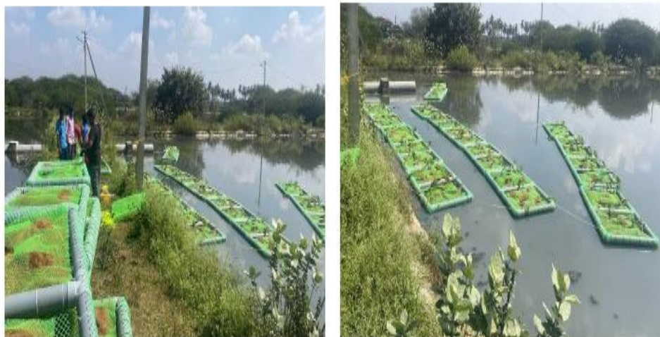
Figure 7: Floating Wetland with Anchorage
