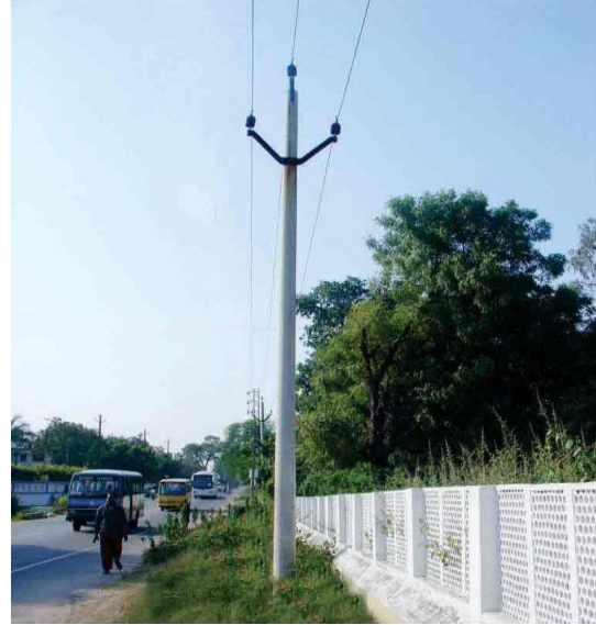
Figure 4: Spun Concrete Pole
