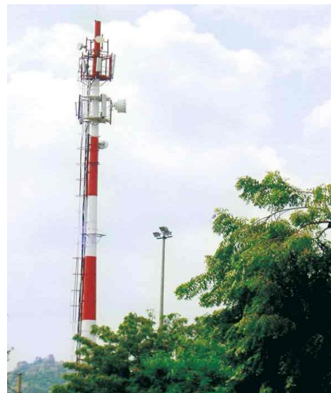
Figure 8: Spun Concrete Tower
