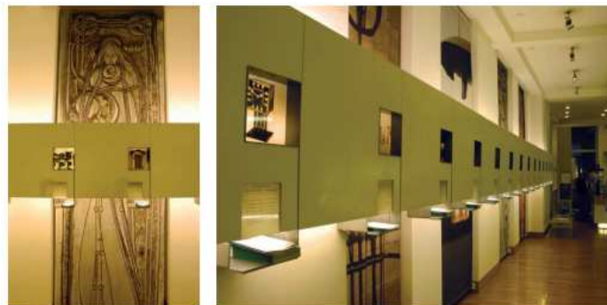
Figure 20: Concealed lighting is mounted within a linear display band. [Source: Lighting for Interior Design]
