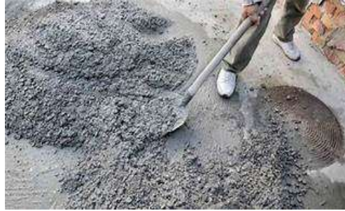
Figure 1: Mixing of the Concrete
