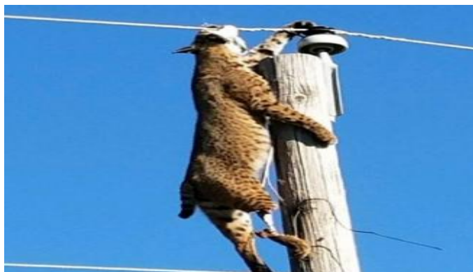
Figure 1: Electrocutation on distribution power lines
