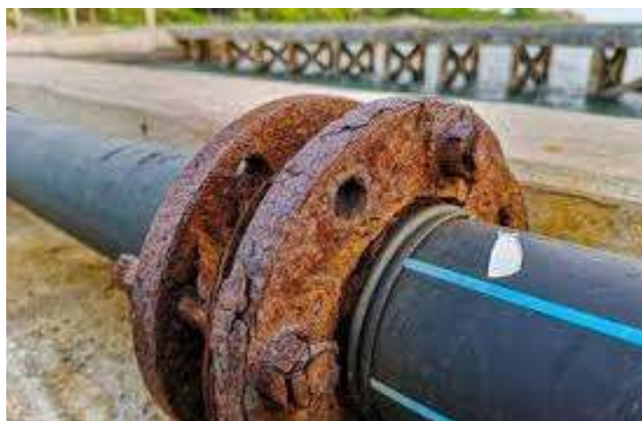
Figure 1: Corroding Pipeline
