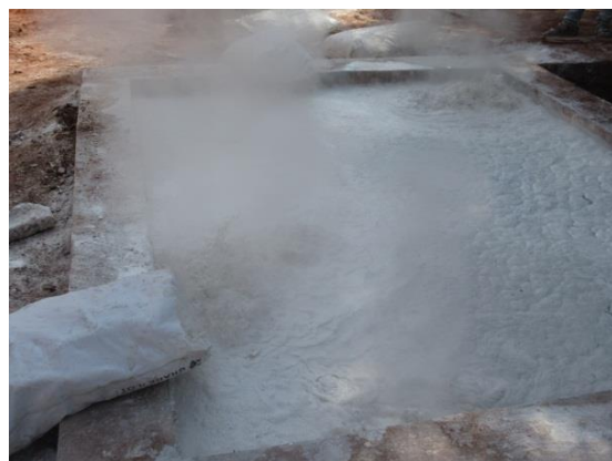
Figure showing the Slaking Process of Lime
