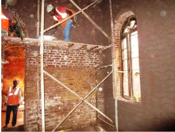
Application of Lime Mortar at site
