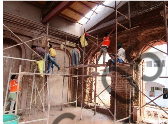
Application of Lime Mortar at site
