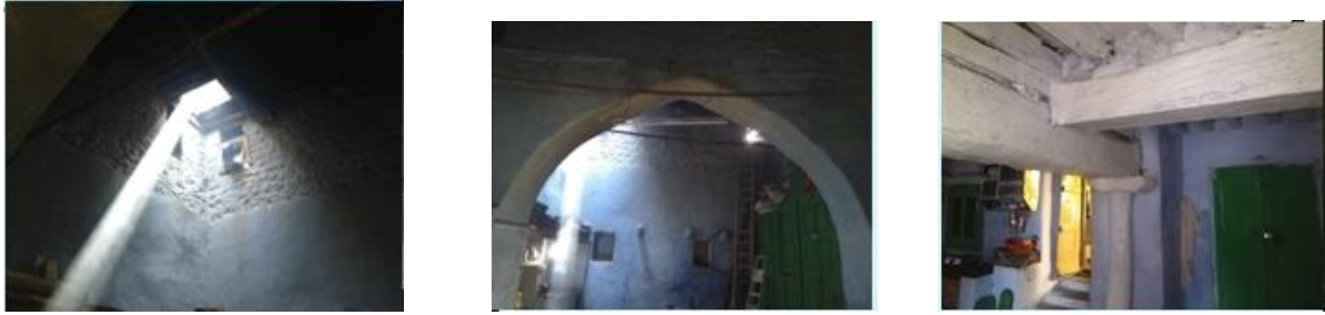
Fig: 29a, b, c (author) Double height kitchen features are same as earlier wada but here surplus amount of light admits through roof ventilators. This wada is bigger.
