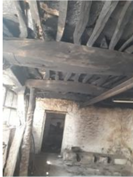
Fig: 19(author) servant's area, Rough finished roof structure.
