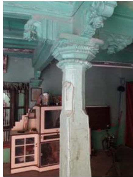
Fig: 16 (author) beautifully carved column & beams
