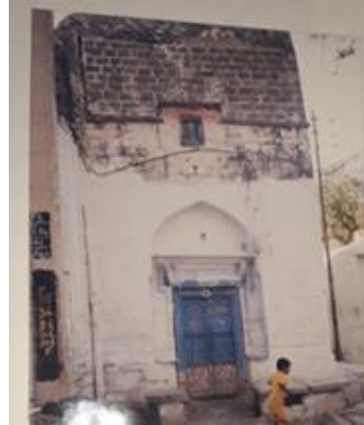
Entrance Door Fig: 12(author)
