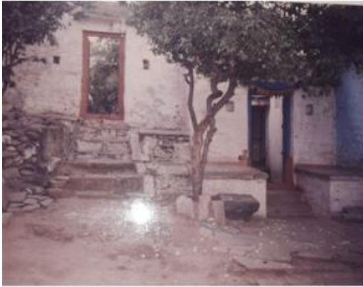
Fig: 8(author) Entrance katta on both the sides with common wall between two houses. Entrance door height and width is also small.
