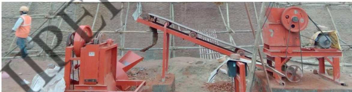
Figure 4: Grinding Machine process of making Surkhi
