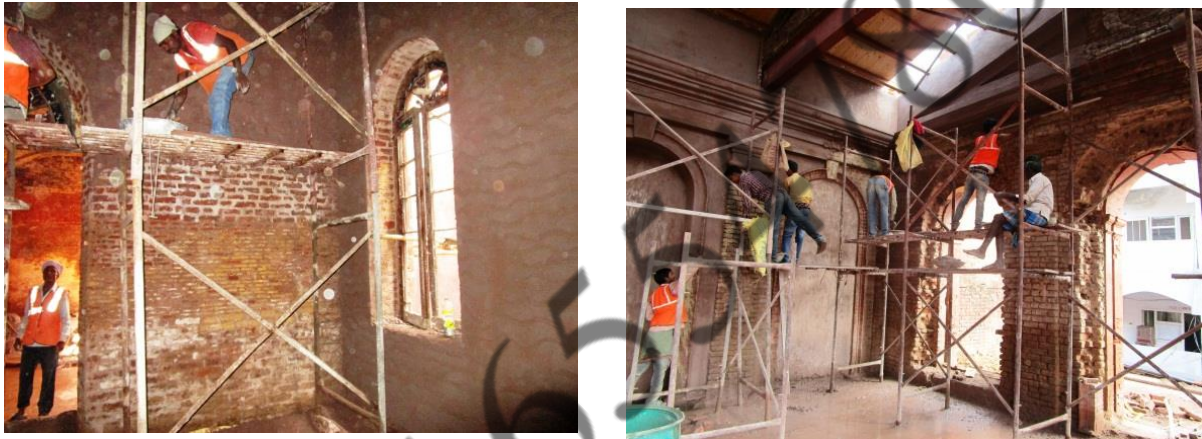
Figure 9: Application of Lime Mortar at Conservation Project
