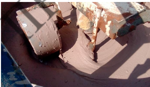
Figure 8: Preparation of lime mortar (1:1:1) - 1 Lime: 1 Surkhi: 1 Sand
