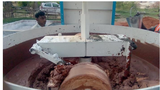
Figure 8: Preparation of lime mortar (1:1:1) - 1 Lime: 1 Surkhi: 1 Sand
