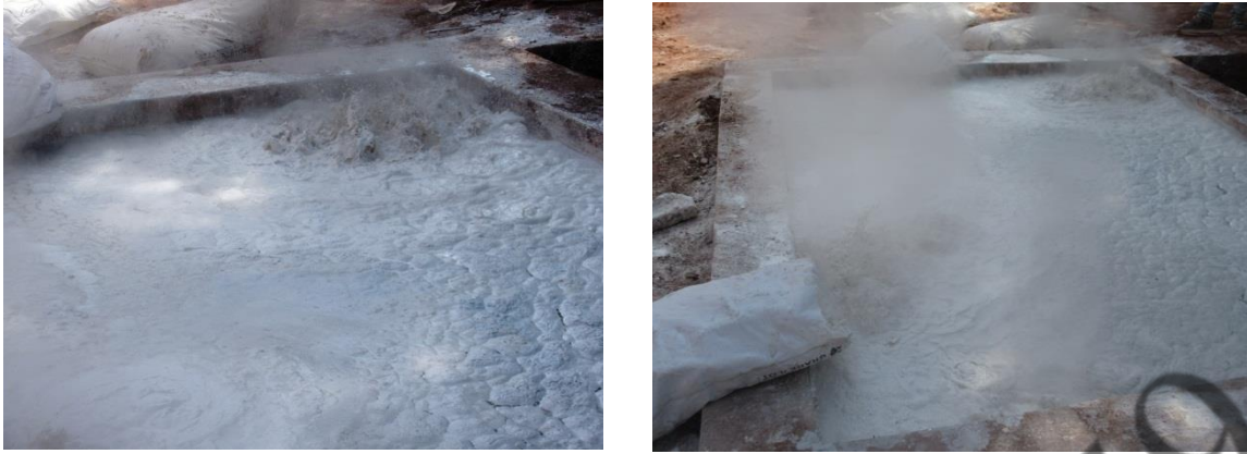
Figure 2: Figure showing the Slacking Process of Lime
