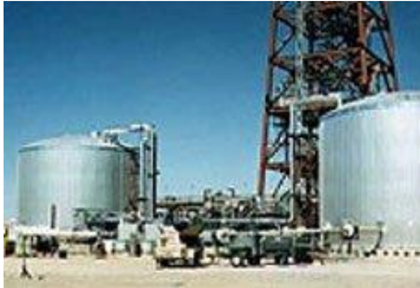
TWO-TANK DIRECT SYSTEM
