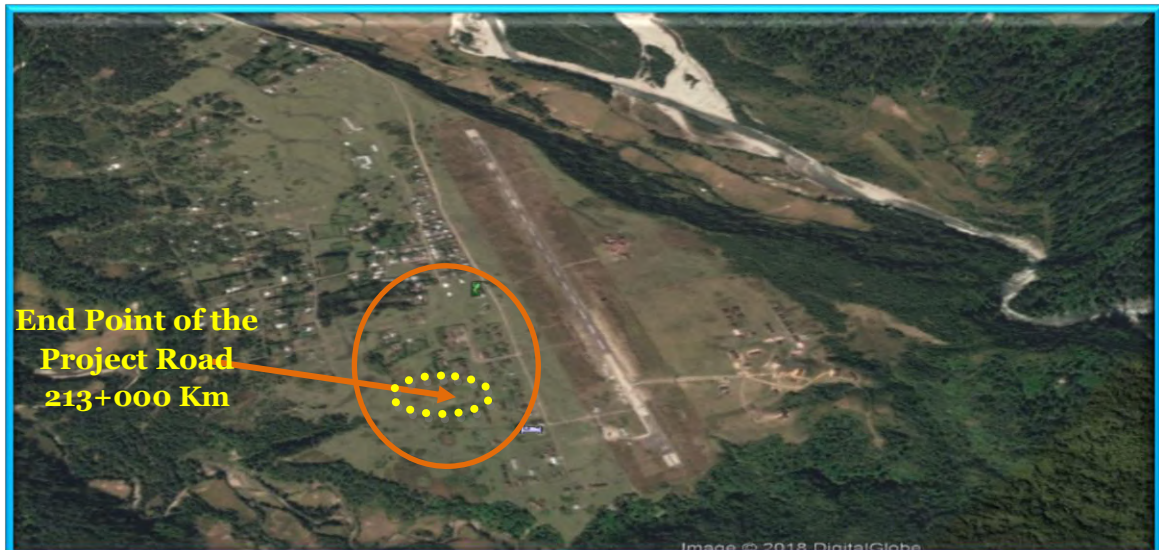
Figure 3 (b): End Point at Vijay Nagar Chainage: 213+000 Km.
