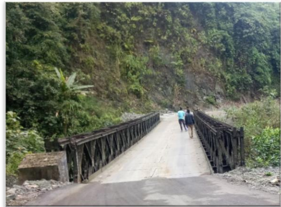
Minor Bridge at Chainage: 108+230.
