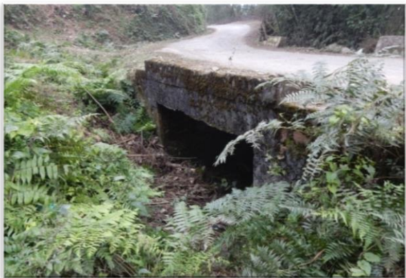
Slab at Chainage: 92+850.
