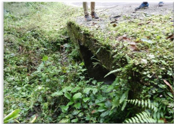
Slab at Chainage: 110+590.
