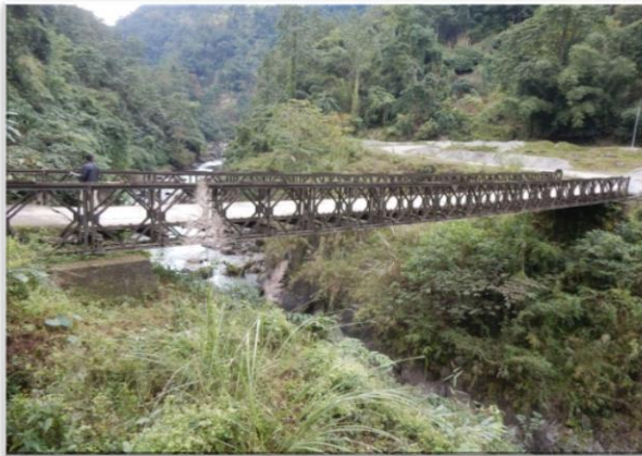
Minor Bridge at Chainage: 101+380.
