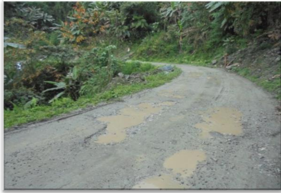
Pavement Existing Condition.
