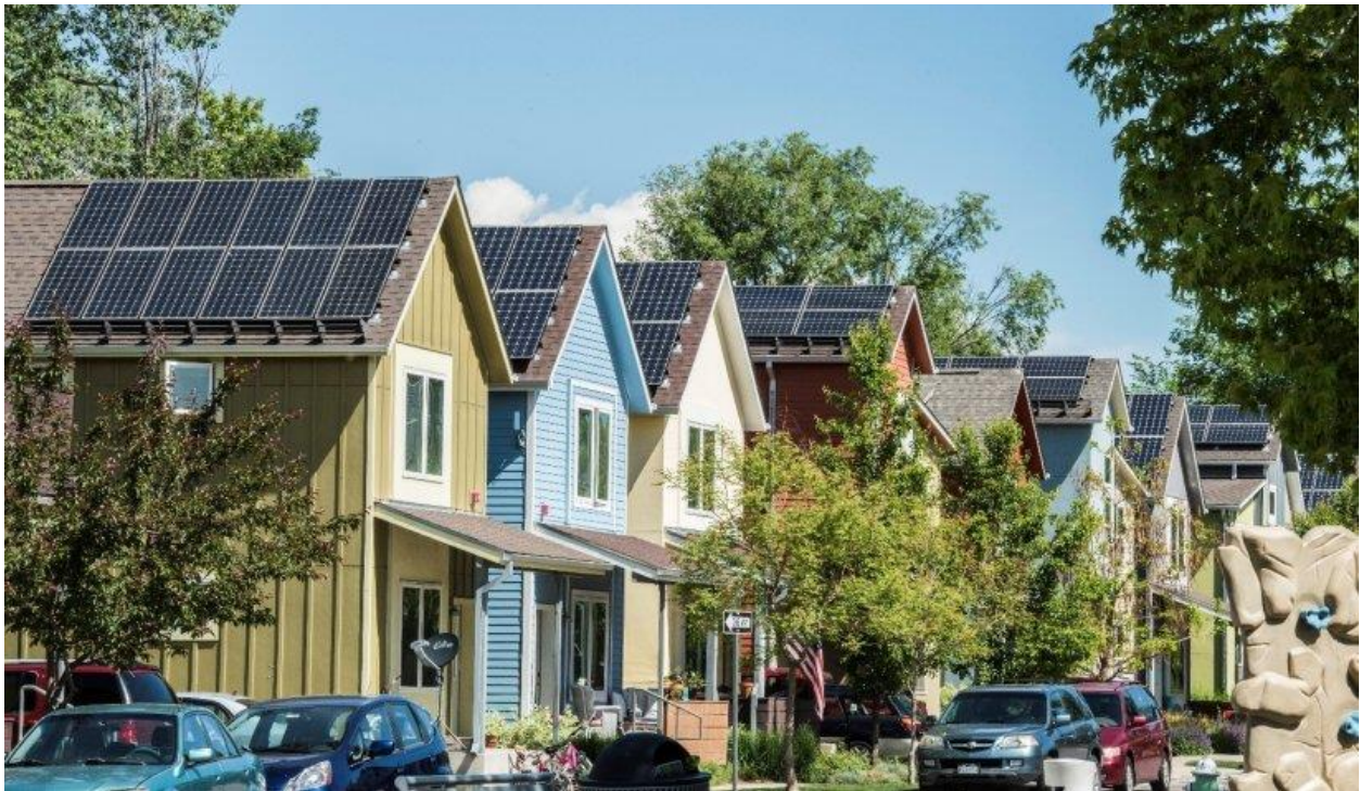
Rooftop photovoltaics in Boulder, CO. Photo by Dennis Schroeder.
