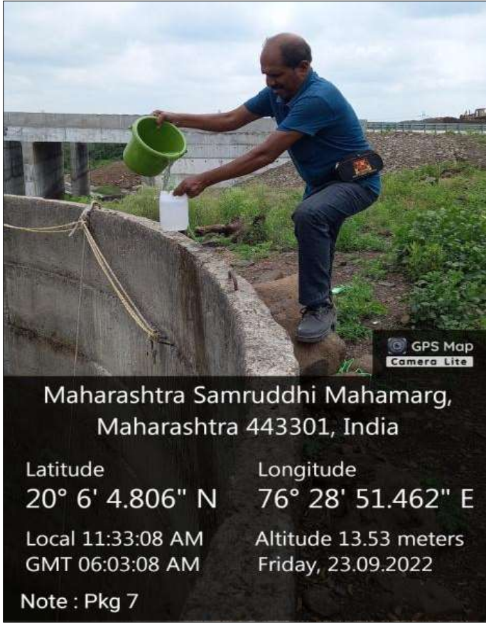
Ground Water (Open Well) Batching Plant @ Km: 297 + 409
