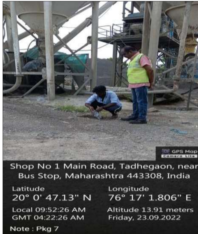
Soil Sample at Base Camp @ Km: 320 + 400
