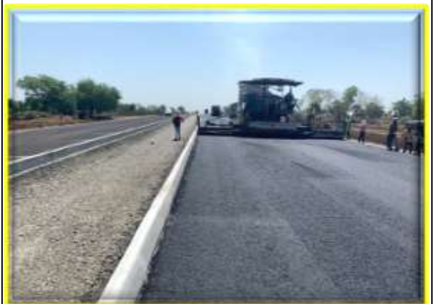
SHREE JI AND ADANI GROUP...!!! Infrastructure India Private Limited Laboratory...!!! AIL Laying in Progress @ Chainage Number 116 + 450 Km to 116 + 750 Km LHS and DBM Laying/ Rolling @ Chainage Number 112 + 300 Km to 112 + 800 Km Setup for Construction along Roads' Network in the Projected Area/ Place/ Camp Site Location.
