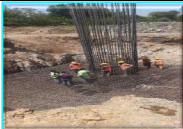
SHREE JI AND ADANI GROUP...!!! Infrastructure India Private Limited Laboratory...!!! Preparation of Foundation and Pier Casting of P - 17 and P - 12 in Progress @ Chainage for Construction along Roads' Network in the Projected Area/ Place/ Camp Site Location.
