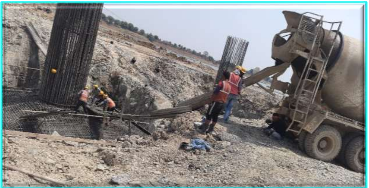
SHREE JI AND ADANI GROUP...!!! Infrastructure India Private Limited Laboratory...!!! Casting of P11 RHS Open Foundation @ Narmada Bridge in Progress @ Chainage for Construction along Roads' Network in the Projected Area/ Place/ Camp Site Location.
