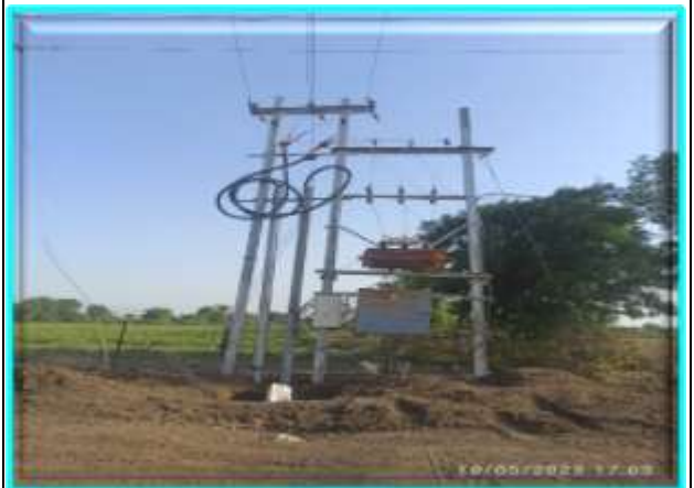
SHREE JI AND ADANI GROUP...!!! Infrastructure India Private Limited Laboratory...!!! AIL Laying in Progress @ Chainage Number 136 + 800 Km to 137 + 360 Km RHS and 200 KVA Transformer Shifting Work Completed with Charger @ Chainage Number 115 + 440 Km near Lela Restaurant Setup for Construction along Roads' Network in the Projected Area/ Place/ Camp Site Location.
