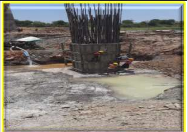
SHREE JI AND ADANI GROUP...!!! Infrastructure India Private Limited Laboratory...!!! Preparation of Foundation and Pier Casting of P - 17 and P - 12 in Progress @ Chainage for Construction along Roads' Network in the Projected Area/ Place/ Camp Site Location.
