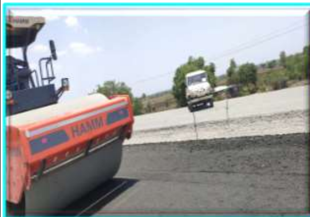
SHREE JI AND ADANI GROUP...!!! Infrastructure India Private Limited Laboratory...!!! AIL Laying in Progress @ Chainage Number 116 + 450 Km to 116 + 750 Km LHS and DBM Laying/ Rolling @ Chainage Number 112 + 300 Km to 112 + 800 Km Setup for Construction along Roads' Network in the Projected Area/ Place/ Camp Site Location.
