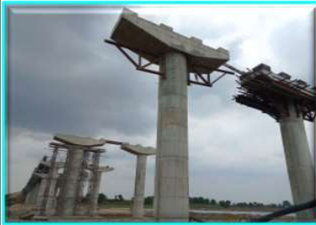
An Imprints of Vertical Pillars Structure Construction Work is Ongoing along Narmada River Side @ Low Flood Level (LFL) Zone...!!! @ Four Laning of Nanasa to Pidgaon Section of NH - 47 (Old NH - 59A) (Indore - Harda, Pkg - III) @ Design Chainage 95 + 000 Km to 142 + 445 Km {Total Designed Length of the Road is = 47.445 Km} @ Projected Site/ Location Chainage.
