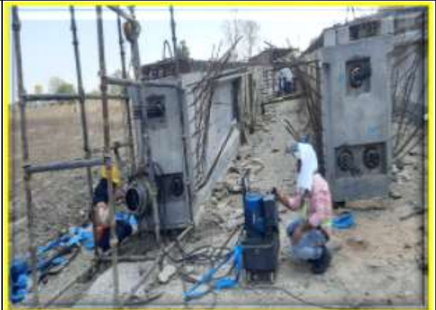
SHREE JI AND ADANI GROUP...!!! Infrastructure India Private Limited Laboratory...!!! Setup for Testing; Measurements; and Analysis of Materials' Strength as well as Weakness like Stressing of PSC Girder @ Chainage Number 110 + 500 MNB...!!! While used in Construction along Roads' Network in the Projected Area/ Place/ Camp Site Location.
