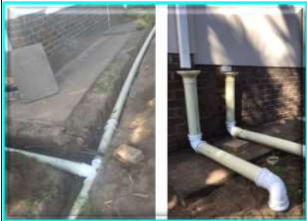
Installing the Pipe System for the Rainwater Collection.
