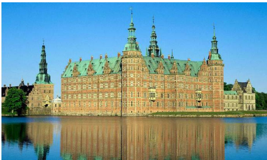
Fig. 3 The Elsinore Castle, Denmark
