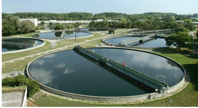
Fig.6: Sewage treatment plant (STP) at OKHLA (New Delhi- India)
