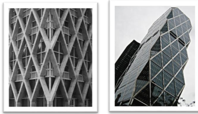
Figure 1 - Example of Diagrid Structural System
