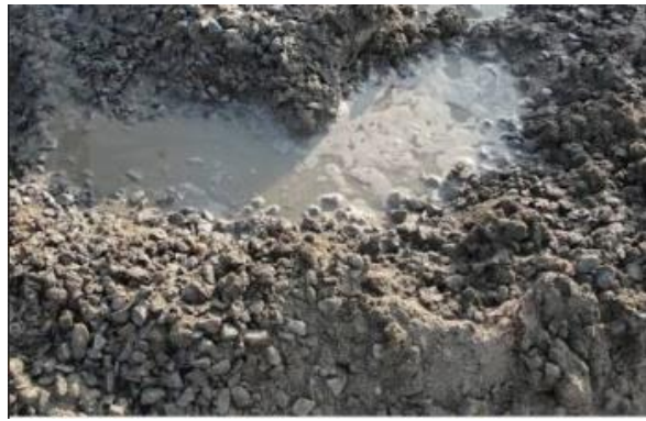
Fig:9 Adding of water
