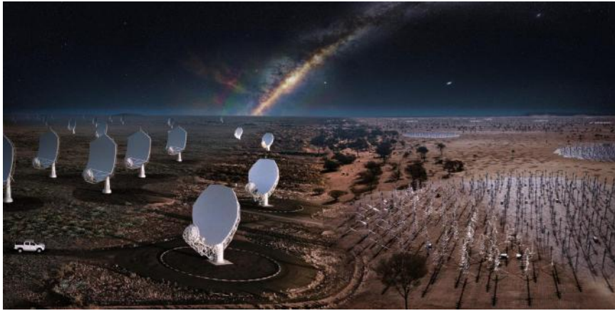
Fig. 4 The Square Kilometre Array: The Square Kilometre Array (SKA) telescope will be the world's largest radio observatory comprising two separate telescopes, SKA-Low and SKA-Mid, constructed in Western Australia and South Africa respectively. In its first phase, The SKA1-LOW telescope will consist of 512 stations of phased dipole antennas spread over a distance of 65 km, and The SKA1-Mid telescope will have 197 dish antennas spread over distances of more than 100 km.
