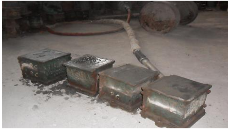
Figure 4. Cement Concrete Cube casting by compaction with Needle Vibrator
