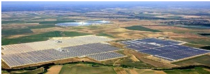
The first three units of Solnova in the foreground, with the two towers of the PS10 and PS20 solar power stations in the background.
